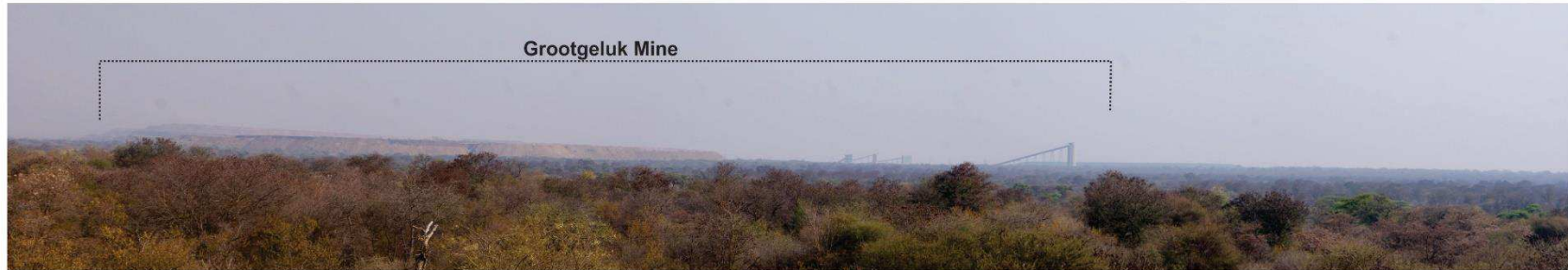
View 9a: View along the D1675 road towards the Grootgeluk Mine
